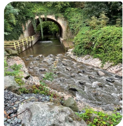
Kingfisher bridge, with fish barrier removed
